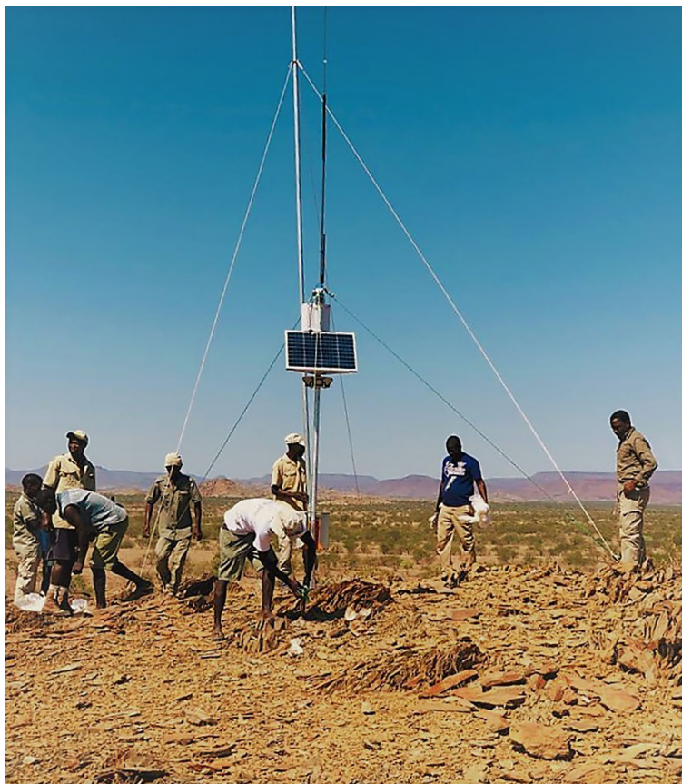
FIGURE 4 Erection of Early-Warning Tower, Anabeb Conservancy, April 2020.
