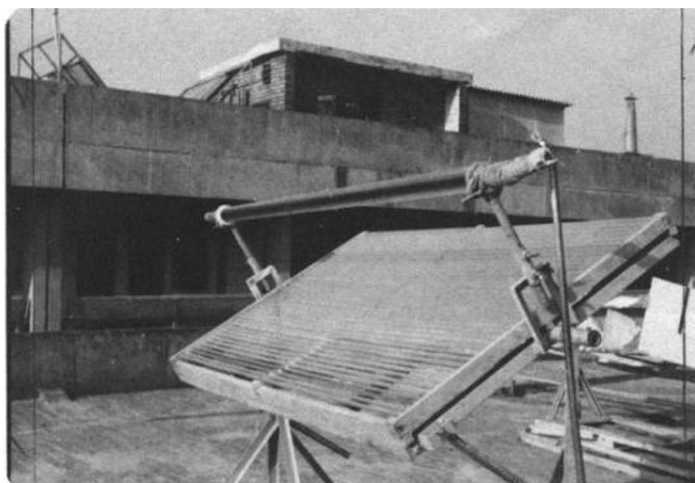
Fig. 4. Tubular receiver without secondary concentrator [39]
