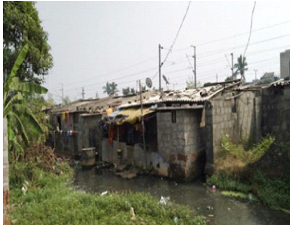
Fig. 3. (a): No proper drainage facilities
