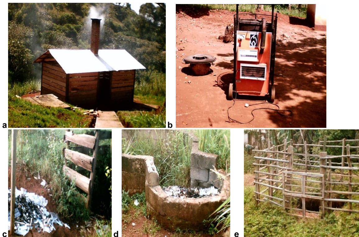
Figure 5. Final waste disposal sites observed in study site: (a) Constructed and fixed Incinerator (b) Mobile incinerator (c and d) Unprotected Medical Waste pits (e) Protected Medical Waste pit.
