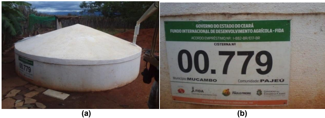
Fig. 5. (a) A Plate cistern in Pajeú and (b) its protection sign Source: Made by the authors (2018)
