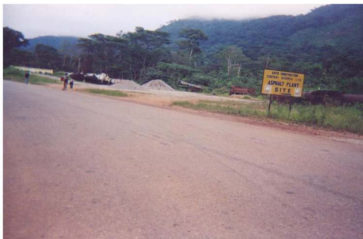
Fig. 5. Asphalt plant of ANFO construction at Kanyang
